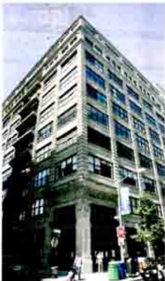
The Gair Buildings, once a manufacturing site for cardboard boxes, reflect the neighborhood's industrial past
